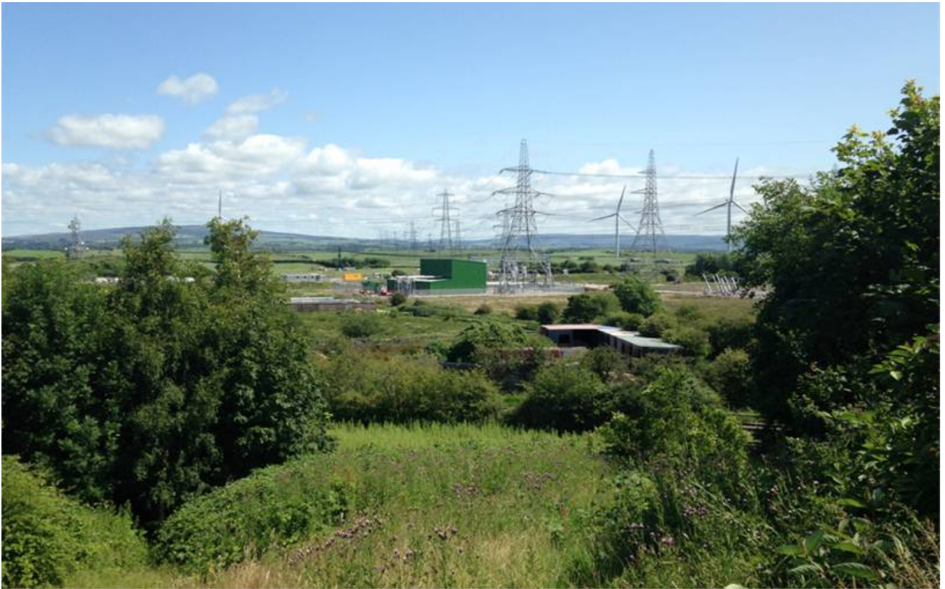
Image 3.5 Existing Middleton 400 kV Substation (Source: National Grid)
