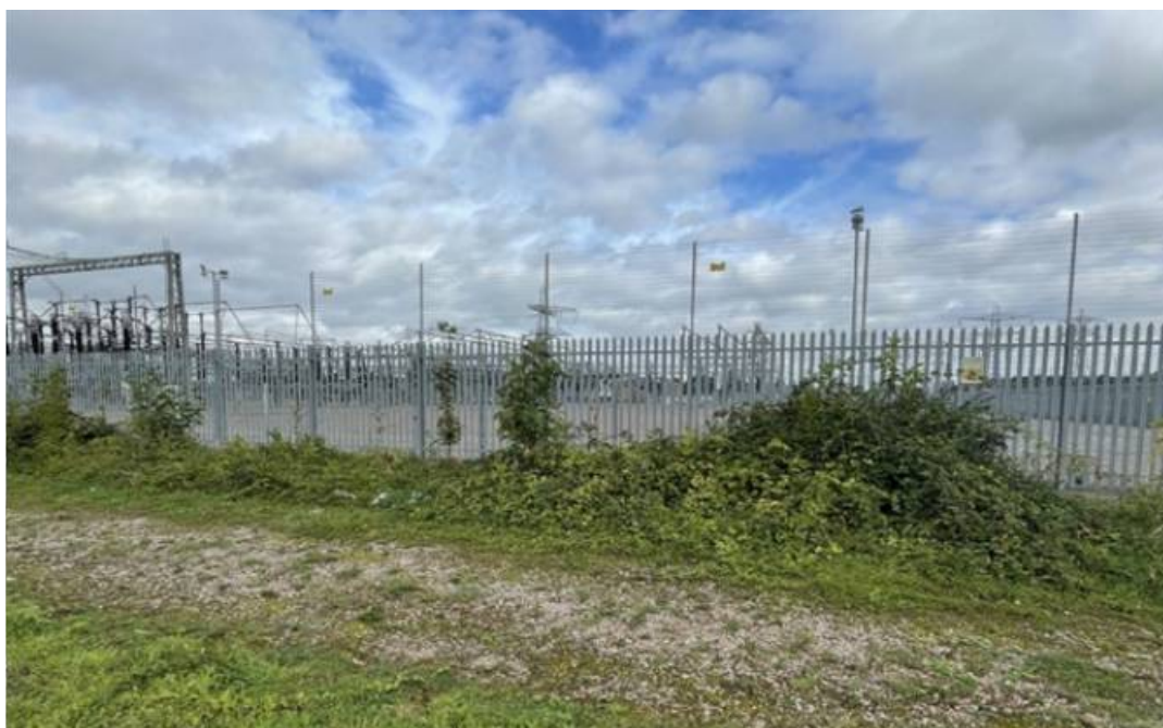
Image 3.10 Existing substation - Norwich Main 400 kV (Source: National Grid)
